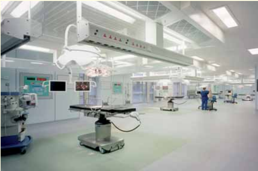
Research suggests that barn theatres, such as this one at Broadgreen Hospital, Liverpool, designed by Nightingale Associates, enhance surgical performance by providing social and professional support to staff
